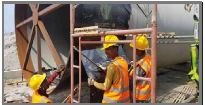
Fig- PipeWrapping 1st Layer at 1320 MW Rampal Power Plant
