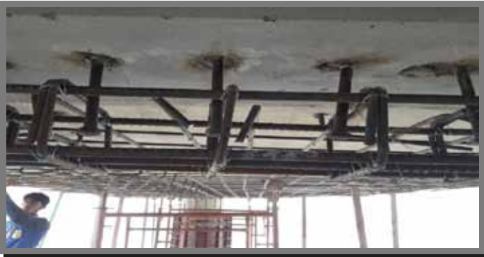
Fig- Bottom Slab Jacketing
