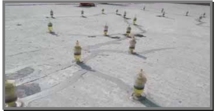
Fig- Crack Sealing by low Viscous Epoxy using ShaliGrout EI
