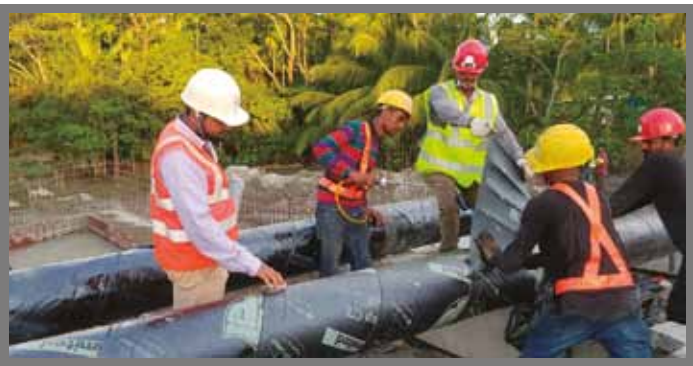
Fig- PipeWrap CT Wrapping at 220 MW Bhola
