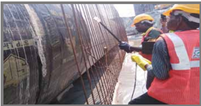
Fig-Holiday Testing PipeWrapping at 1320 MW Rampal Power Plant
