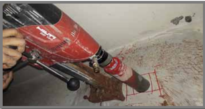
Fig-Concrete Core Cutting
