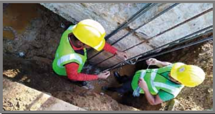
Fig-Retrofitting Below grade beam
