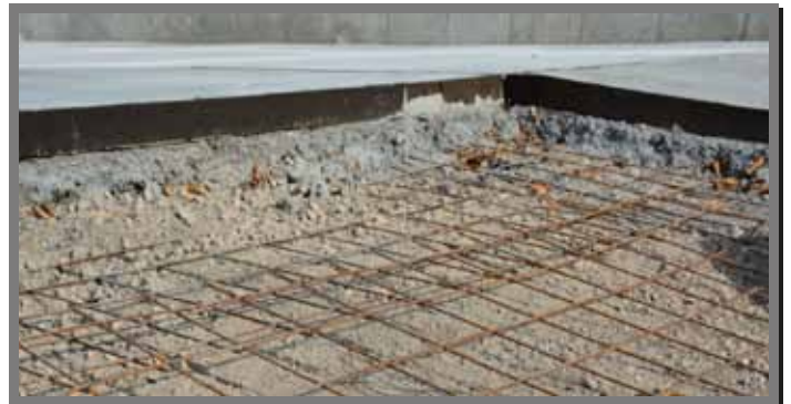
Fig- Concrete Expansion Joints (Shalitek Joint Filler Board)
