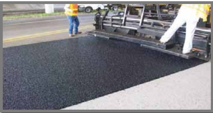
Fig- ShaliSeal RS TC Road Emulsion (Top Coat Road Slurry for Enhancing Road Life by Preventing Water Ingress
