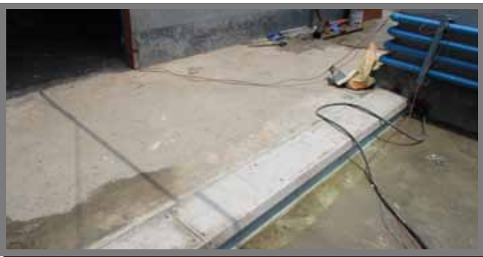
Fig-Aluminium Angle for Expansion Joint
