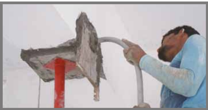
Fig-Grout Pumping at Beam Void Filled
