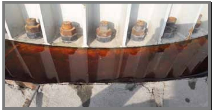
Fig-Epoxy Grouting using ShaliGrout EI
