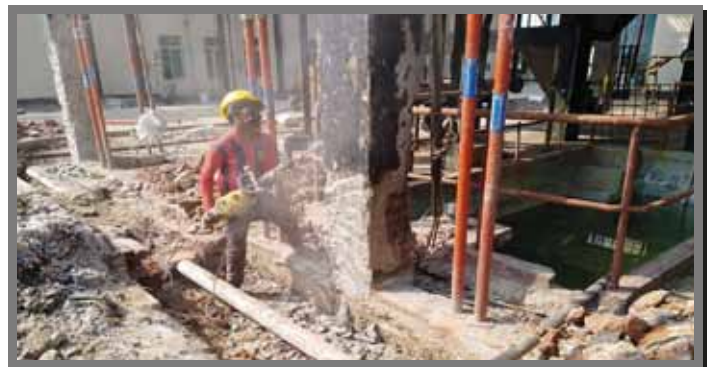
Fig-Removal of Plaster & Loose Concrete
