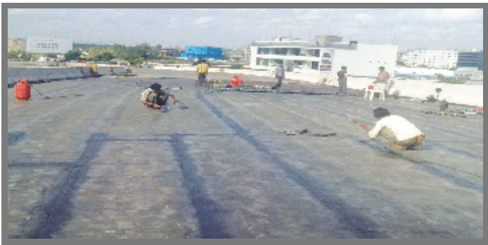
Fig- App Modified Waterproofing Mebrane using SuperThermolay
