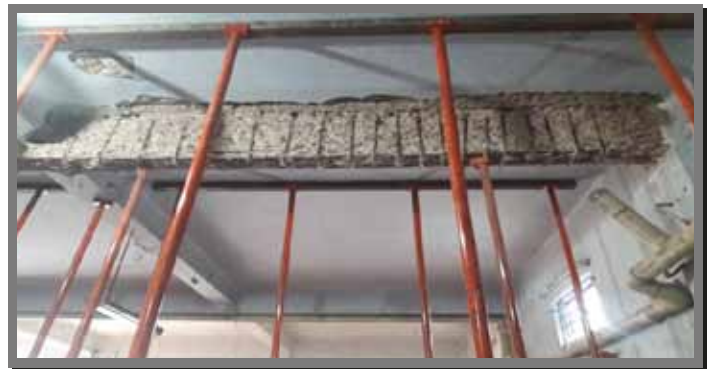
Fig-Beam Retrofitting
