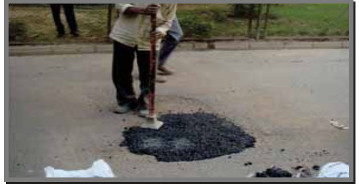
Fig- Instant, Convenient & Durable System to Repair Pot-Holes (ShaliPatch)
