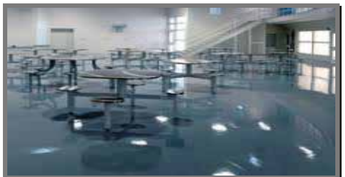
Fig- Self Levelling Epoxy Floor
