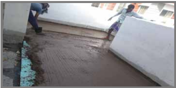
Fig- Thermal Insulation Board With CC Casting
