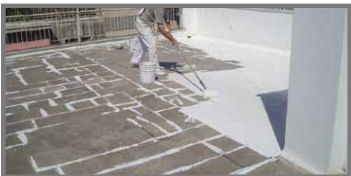
Fig- Waterproofing by PU Liqueid Membrane Without Removal Tiles
