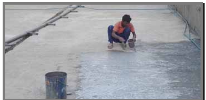
Fig- WP Prime Coat at Sheraton Hotel
