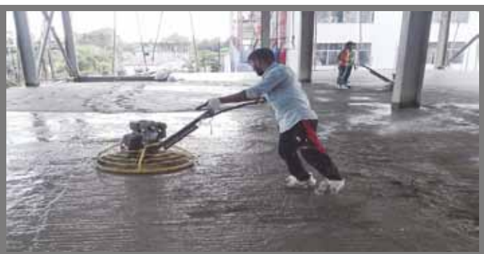
Fig- Floor Hardening Using Power Trowel Machine
